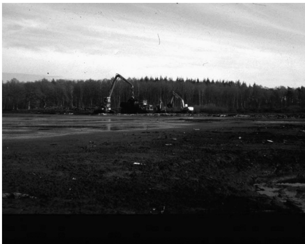
Figure 2. Drainage of the Venkoelen during restoration activities (removal of degraded sediment to a depot).
